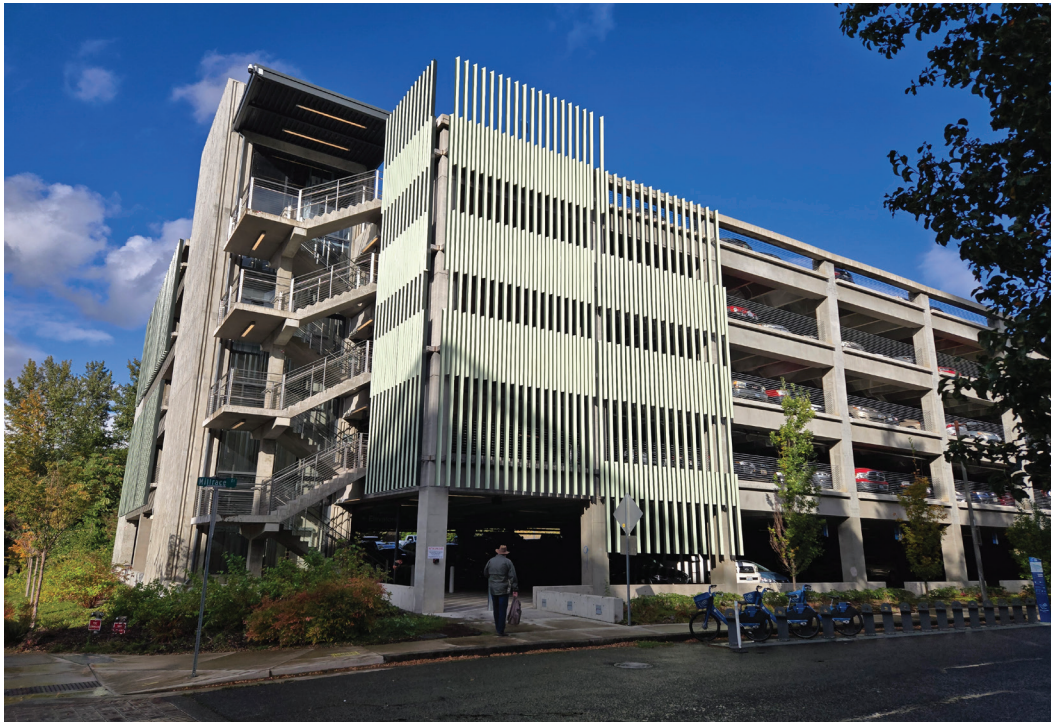
Millrace Parking Garage
