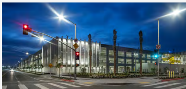
LAX ECONOMY PARKING STRUCTURE, LOS ANGELES, CA (KPFF)
