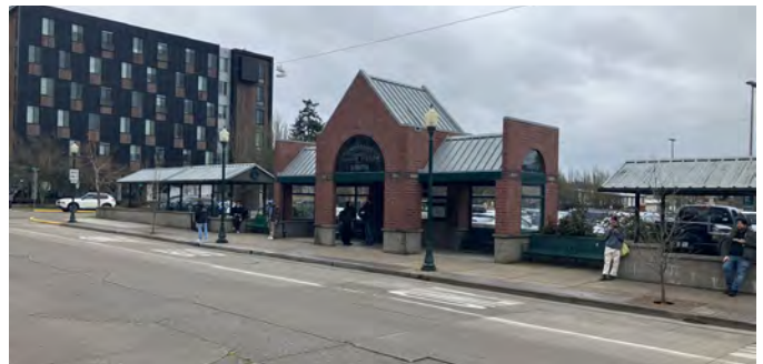
SITE C - PLC LOT
