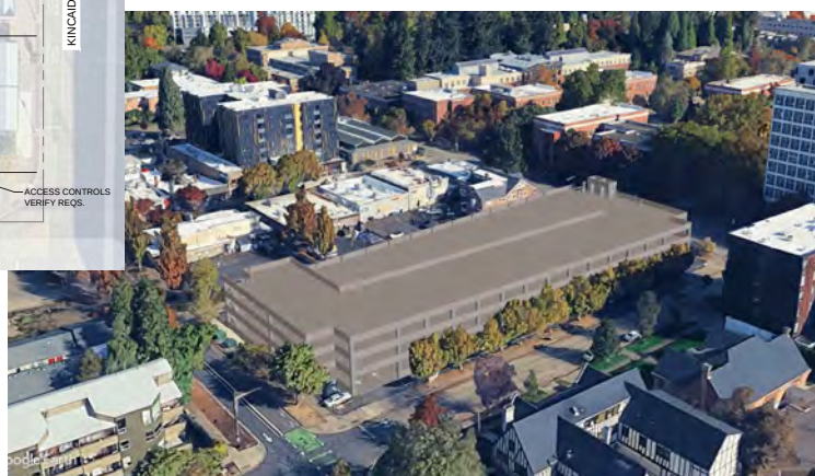
SITE C - PLC LOT
